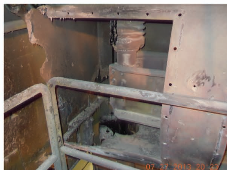
A WORKER INSPECTS THE FAULTED ISOLATED PHASE BUS. PHOTOS COURTESY AMEREN MISSOURI.
