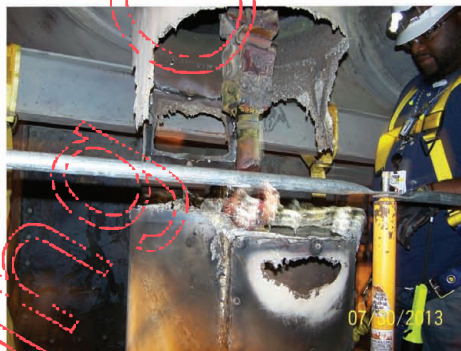
A WORKER INSPECTS THE FAULTED ISOLATED PHASE BUS. PHOTOS COURTESY AMEREN MISSOURI.
